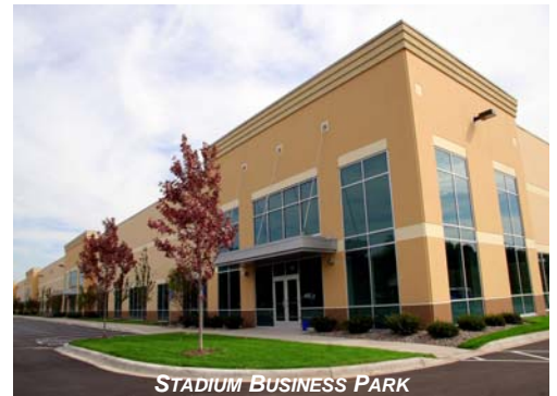
STADIUM BUSINESS PARK
