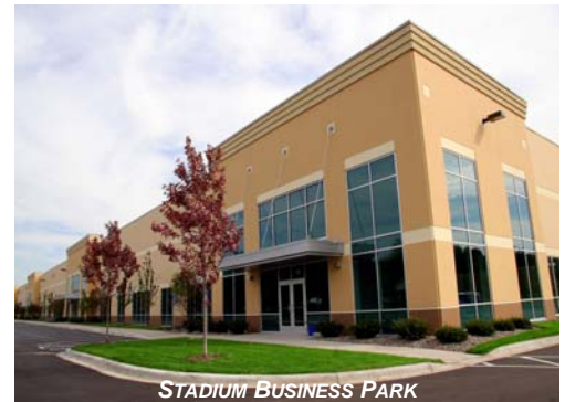
STADIUM BUSINESS PARK
